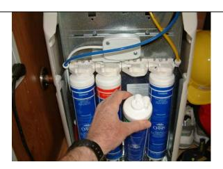
Step 7 Remove the two rubber seals on the top of the new cartridge that is to be installed.
