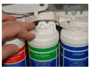
Step 6 Pull the top of the cartridge towards you to remove it. The cartridge will pivot on its bottom. Lift the used cartridge up and out.
